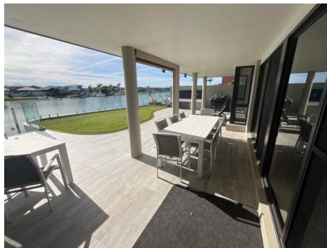
Photo Ref #36: The patio is in fair
