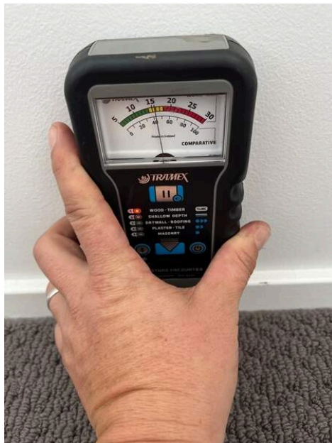
Photo Ref #18: There are higher than average moisture readings to the bedroom four front wall. This will require further investigation to ascertain the origin of the readings.
